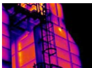
Petrochemical & chemical industries
